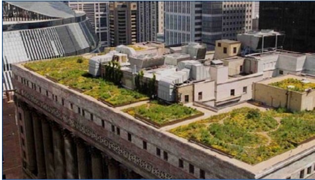
Green roof in Chicago
