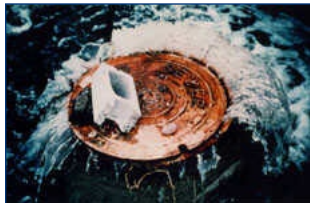
Rain can overload sewers
