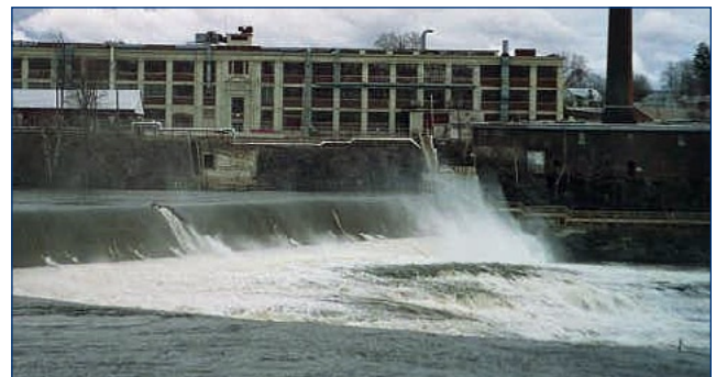
General Electric plant at Hudson Falls, N.Y.
