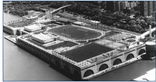
New York City's North River Treatment Plant
