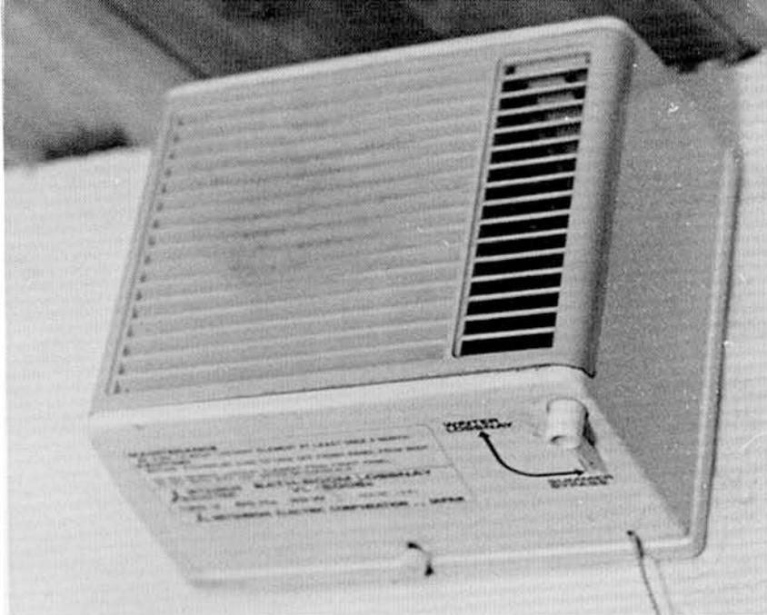
An 18-inch-wide air-to-air heat exchanger mounted in the Lovinses' bathroom.
