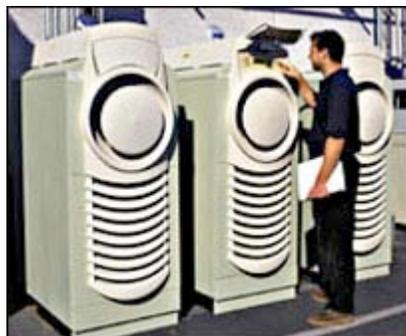
Microturbines work like natural gas-powered jet engines but produce electricity instead of thrust.
